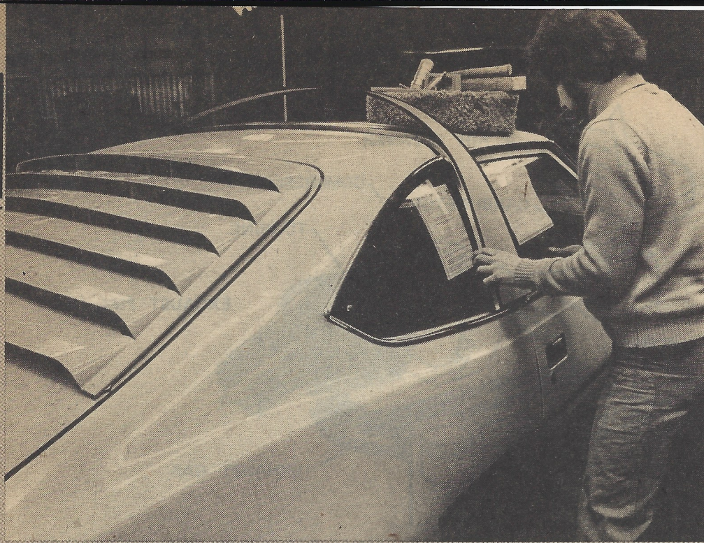
The brushed aluminum Targa style band being installed on a Hornet AMX at the Motortown facility in Wisconsin. Note the rear window hinged louvers already in place, also done by Motortown.
